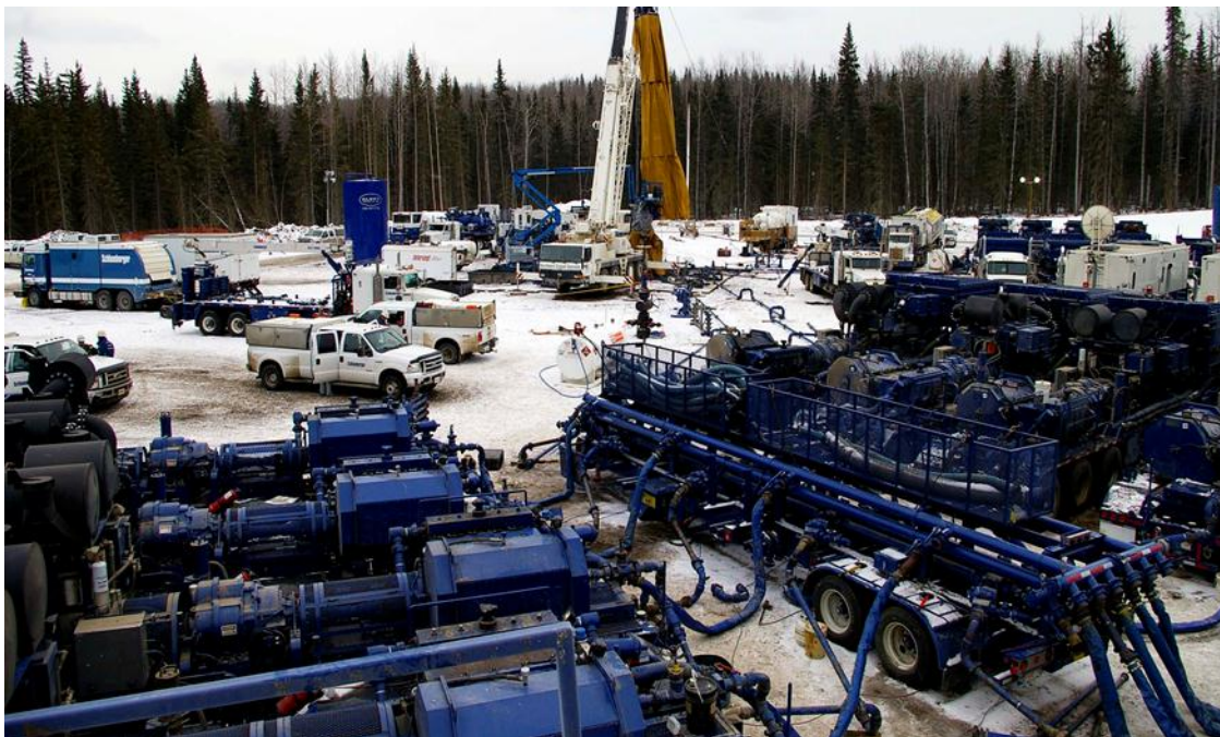
Slickwater Frac underway – Montney Shale - source: Talisman Energy Polska Sp. z o.o.
